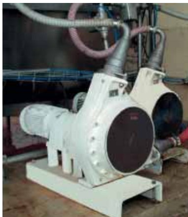
Z pump in transfer of poultry blood
