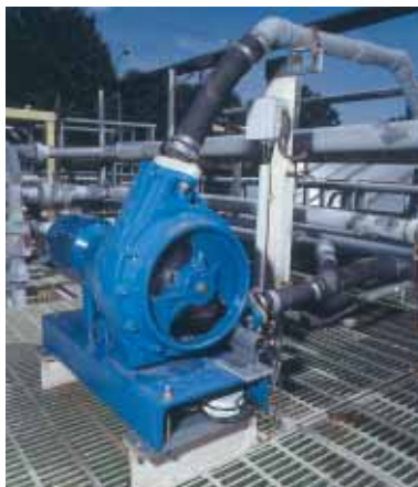
Z pump in neutralization of effluents
