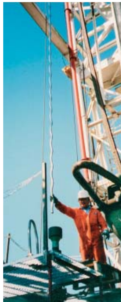
Installation of the PCP. Running in the rotor
