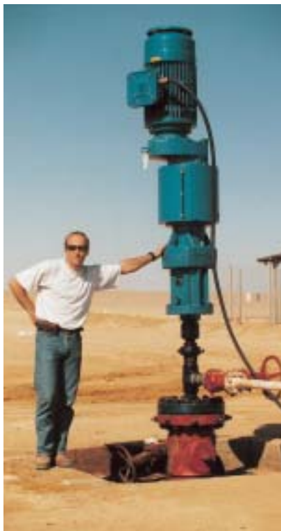
Commissioning a PCP in Libya (Drivehead VS 60 HP with moto-reducer)
